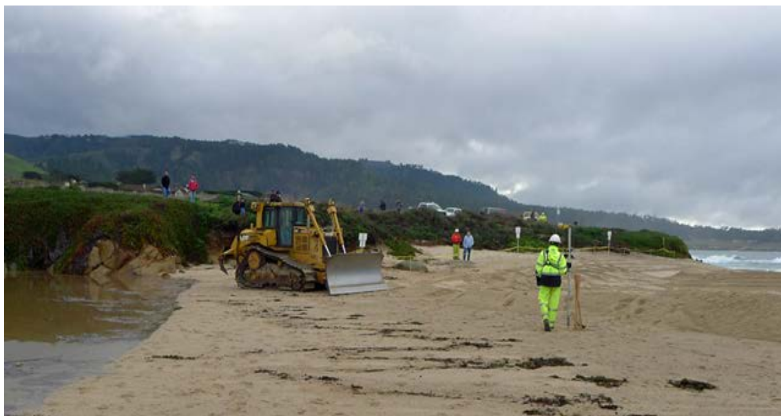
County crews at work at the Carmel Lagoon.
