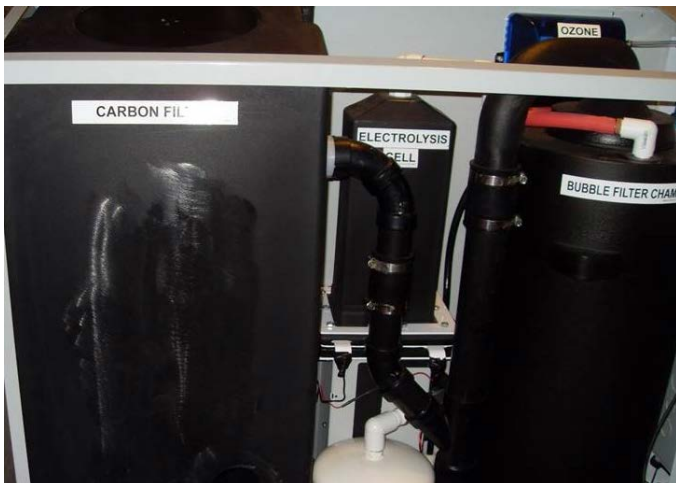
Gray water system components in place both inside and outside of the home (above and at left).
